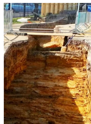
The trenches around the site are getting bigger
